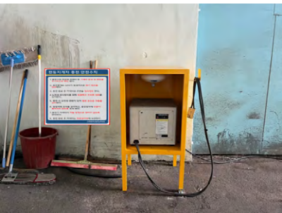
Installing forklift charging station
